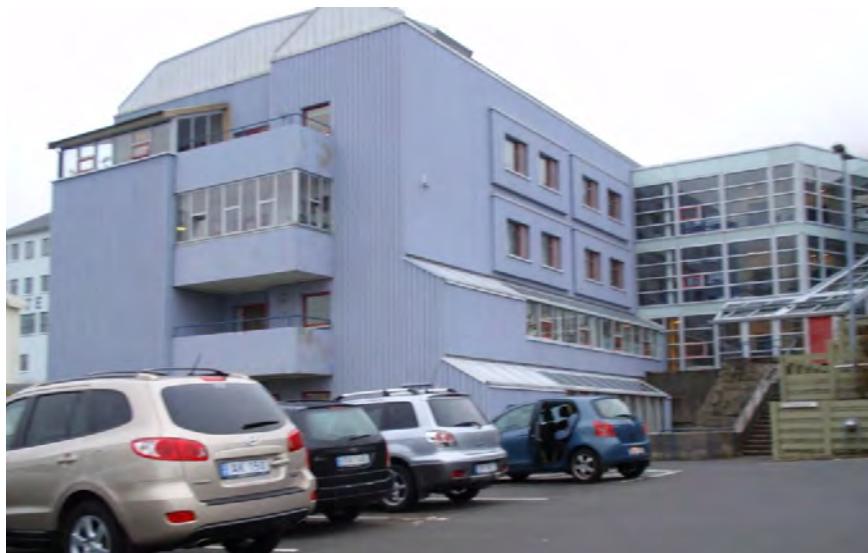
Figure 3. Klaksvik Hospital. The sewage line was accessed through a manhole at the parking lot
